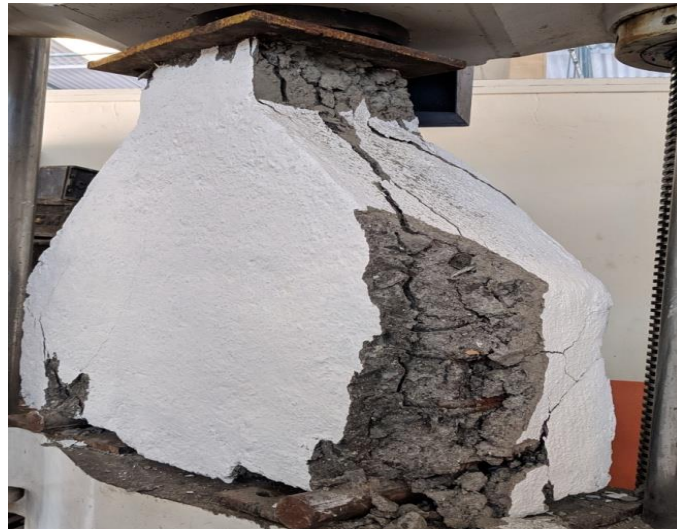
Fig.5. Crushing of compression zone of corbel.
