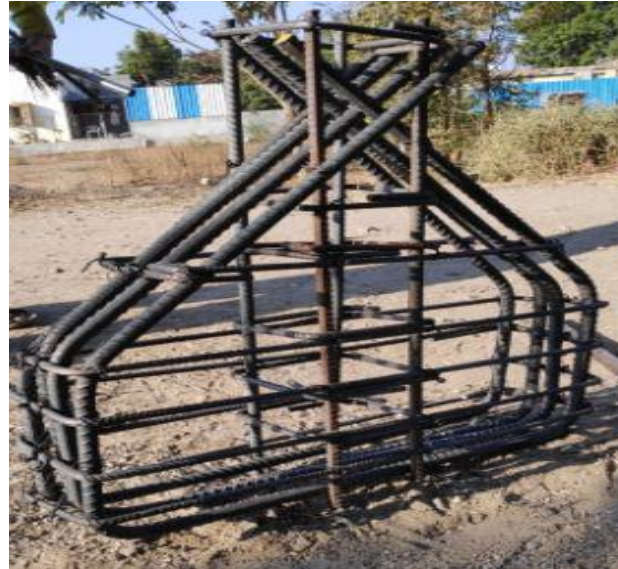
Fig.2. Reinforcement of corbel.
